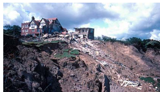
Devastation caused by landslides
